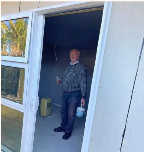
Jim Bhai finishing the room
