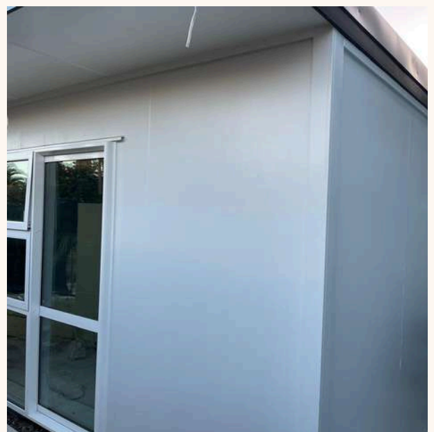
Completed guest room
